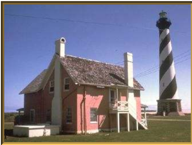
"Cape Hatteras National Seashore (North Carolina)" by National Park Service
